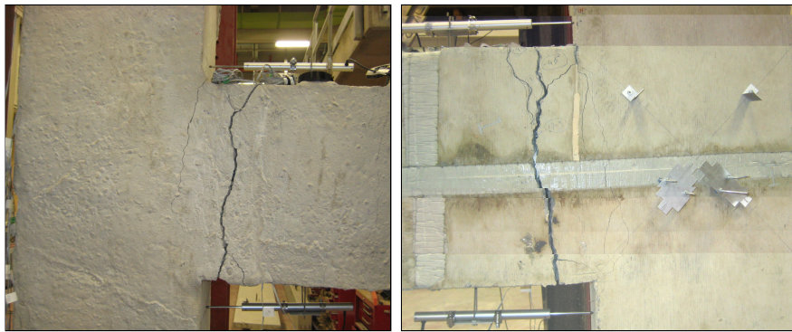
Fig. 14. Crack pattern of specimen JBC-4 after being subjected to cycles up to 4.4% drift (a) front face, and (b) rear face.
